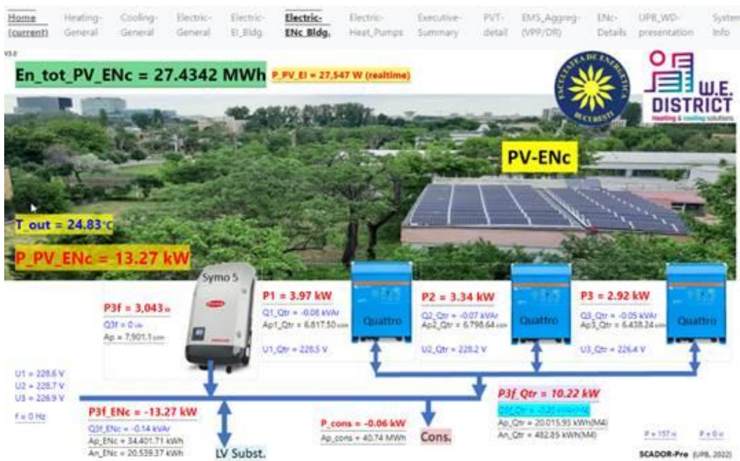
Figure 81. Second PV system in NUSTPB (26 kW).
