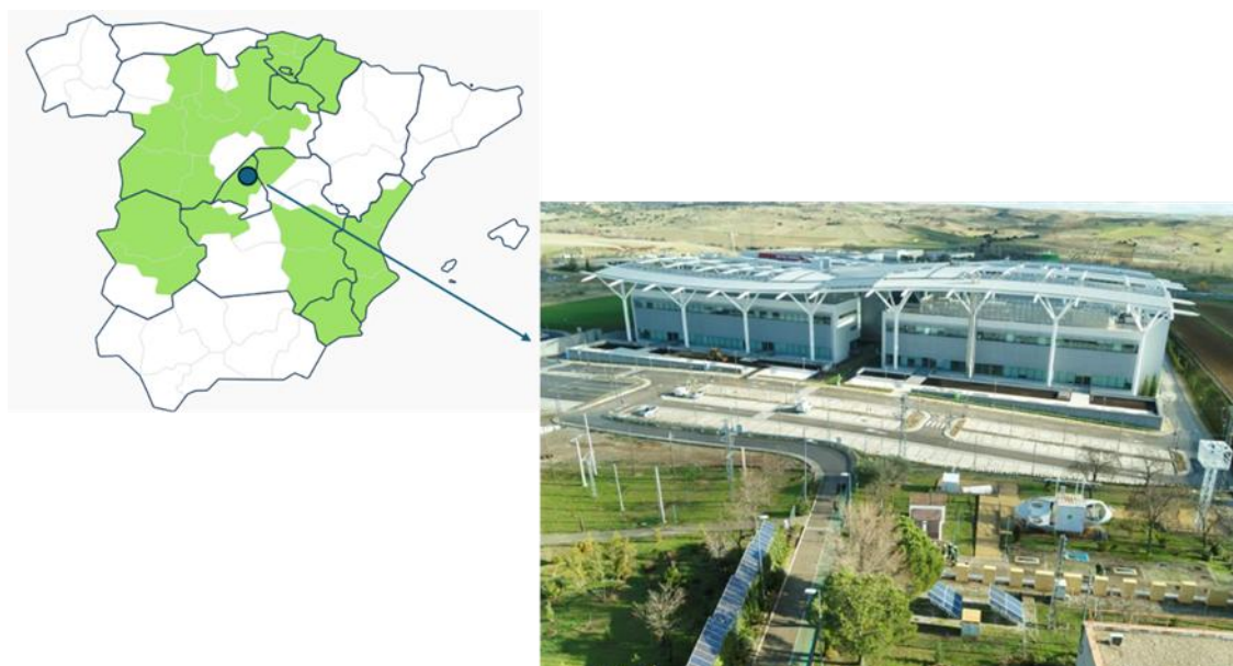
Figure 84. Spanish demo site. In the left, in green it is represented the distribution area from i-DE in Spain. In the right, an image of the Iberdrola Campus located in San Agustín de Guadalix (Madrid).
